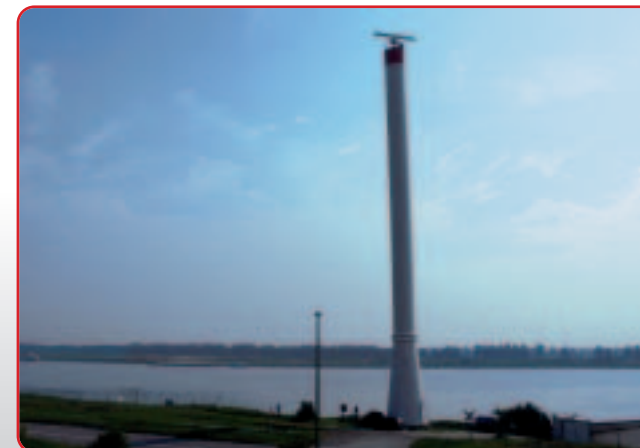
Radar antenna of VTS Antwerpen
