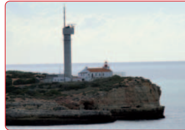
Radar antenna of VTS Portugal
